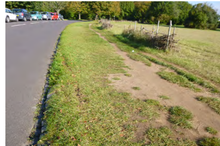
Erosion of the grass areas where there are informal running/walking routes alongside the road edges and inside the avenues of trees
