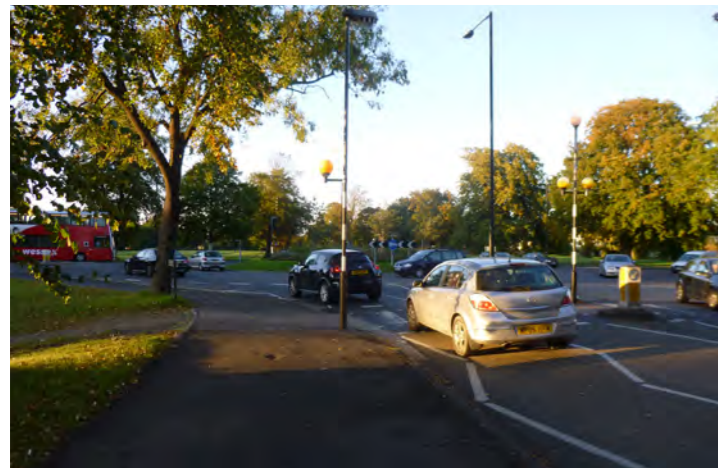
Road junctions and roundabouts which have poor connectivity with a lack of crossing points and pathways on one side of the highway. This is difficult for pedestrians and cyclists to use
