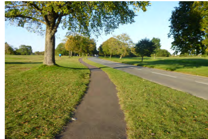
Historical narrow bitmac path routes, with a grass verge area separating the pedestrians from the road traffic.
