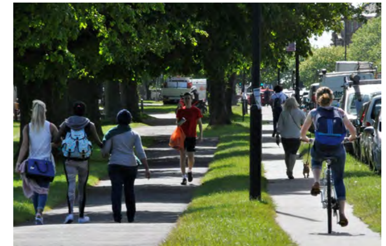
Poor legibility of the existing segregated cycle provision along Stoke Road leads to uncertainty for both pedestrians and cyclists
