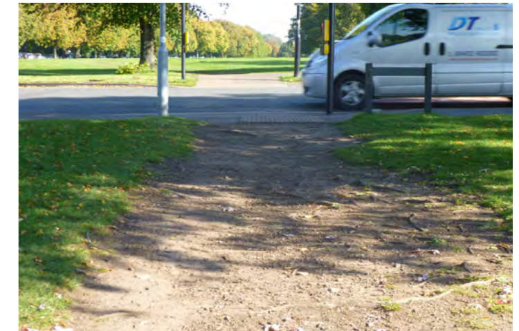
Erosion of grass areas at key crossing reflects the poor connectivity with adjoining routes, the high levels of foot traffic, and the desire lines of visitors enjoying The Downs
